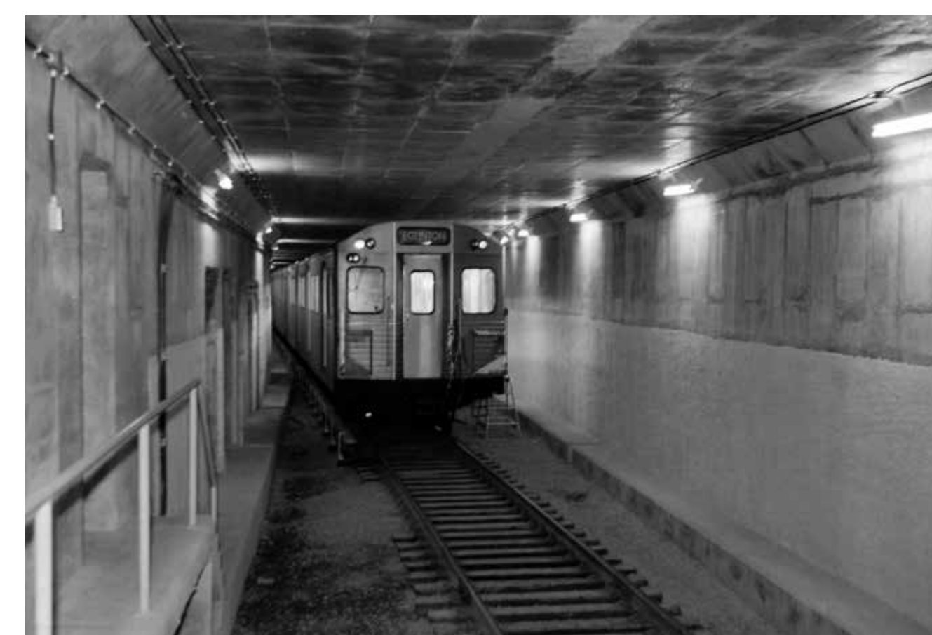
Previous track design consisted of wooden ties on a gravel bed.
