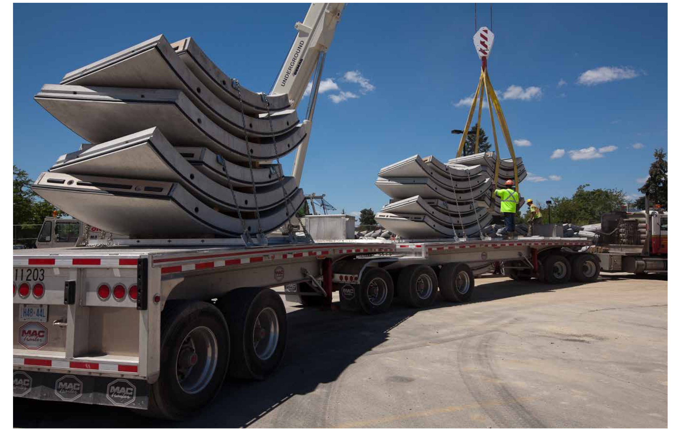
Delivery of Tunnel Liners
