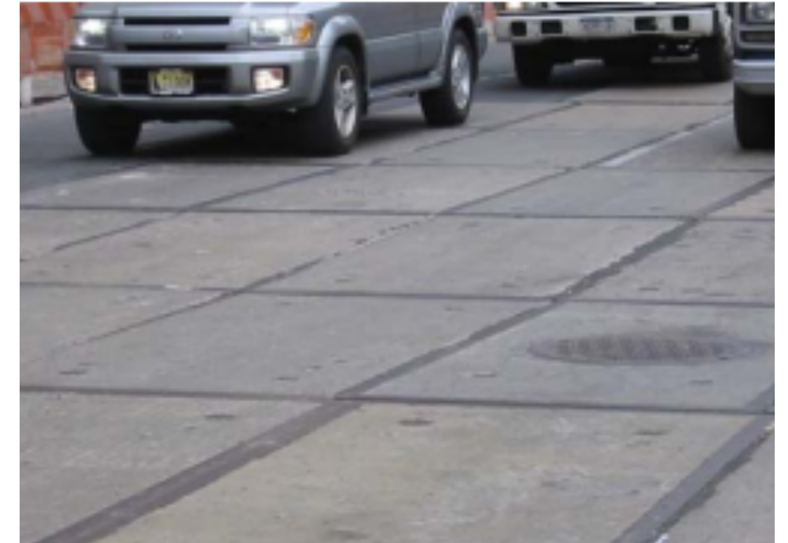
Example of decking above construction area – allows for near normal traffic operations
