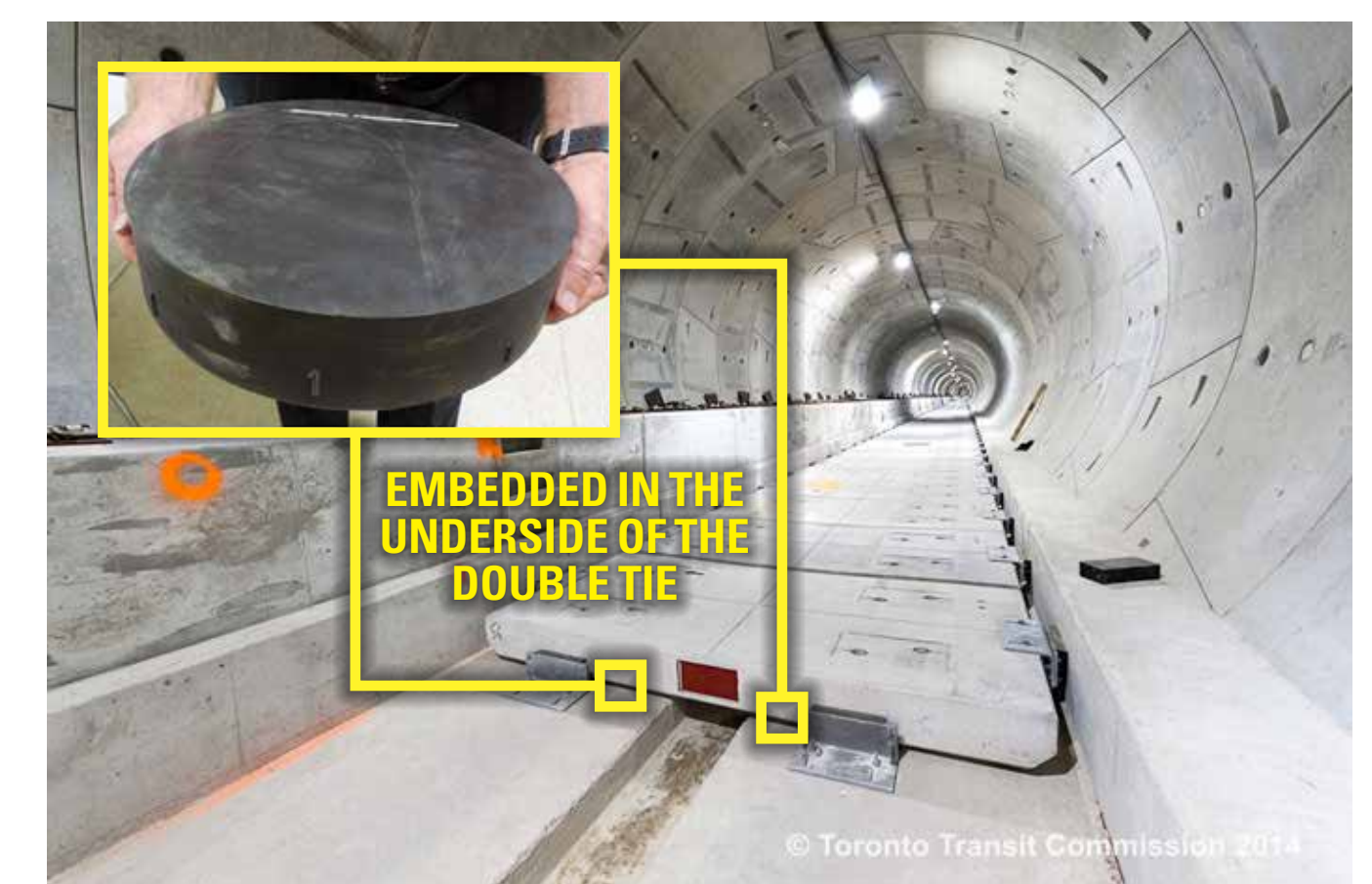
Contemporary track design consists of double ties with rubber pads known as Isolation Pucks.
